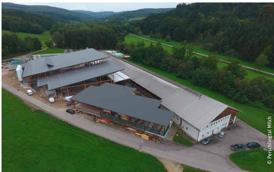
Barn facility for 365 dairy cows
