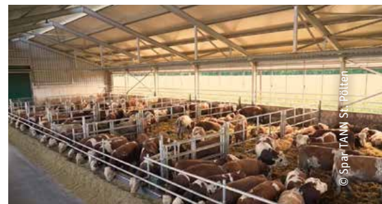
Cubicle barn with paved floor, a manure scraper in the feeding area and litter bedding
